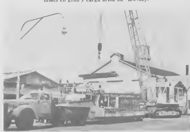
ON THIS spot above, Lago's cold storage building stood for thirty-one years. Slabs from ceiling and walls were lifted by a mobile crane and loaded on a low-boy. They may be dumped later on the harbor reef. E LUGAR aki tabata e sitio camina e edificio di Cold Storage tabata durante treinta y un aña. Planchan di plafon y mura y a worde lamá cu grua y cargá riba un "low-boy."
